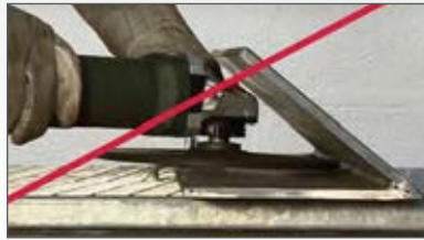
This solution violates safety standards
